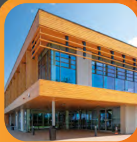
The Bridge Leisure Centre
